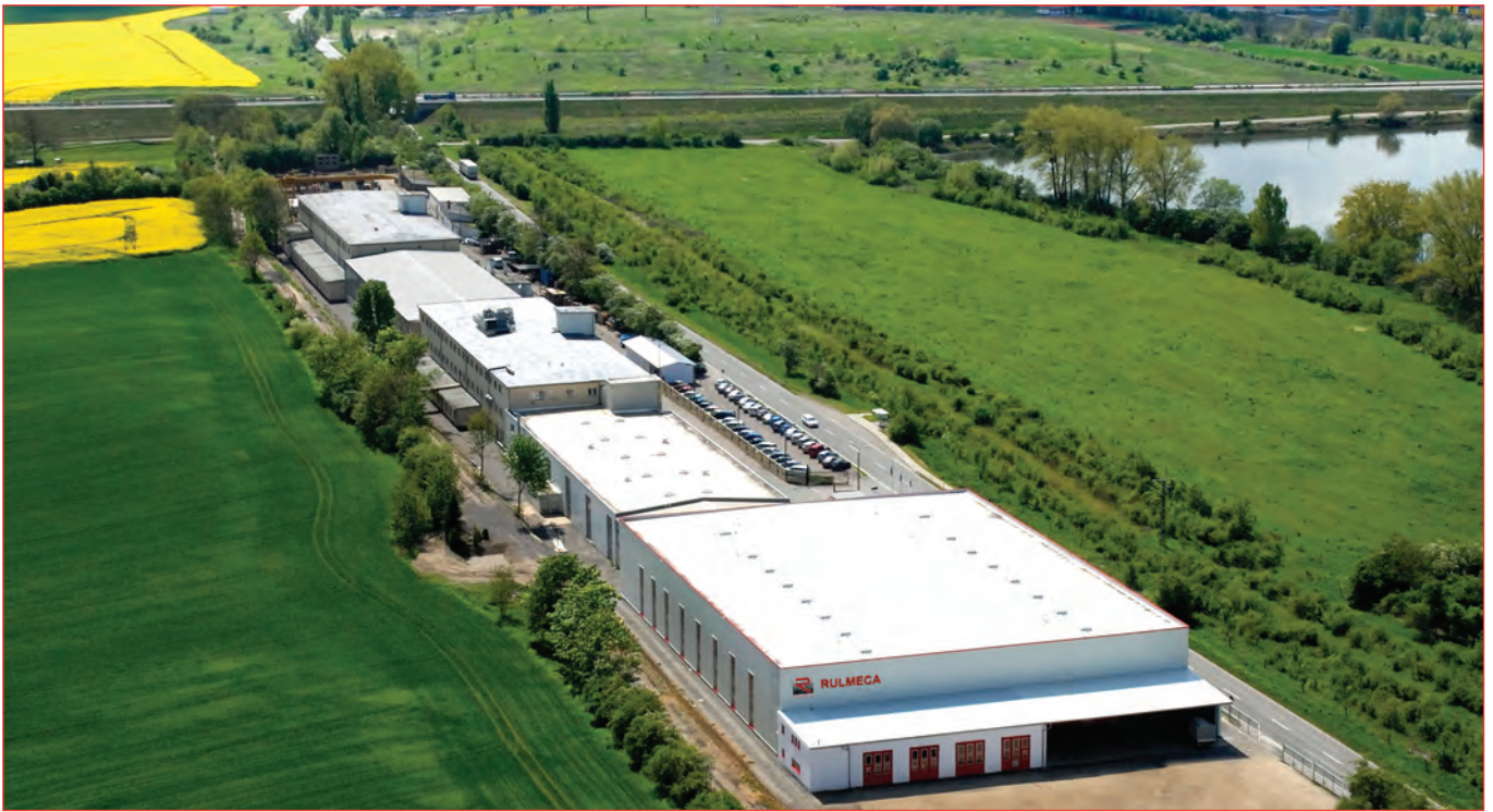
RULMECA GERMANY GmbH, Aschersleben, Germany - Rulmeca Motorized Pulley Manufacturing Facility.
